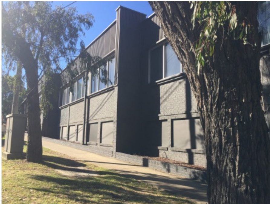
Photo 5.1.1 View of northern side of building on site, adjacent to Ella Street
