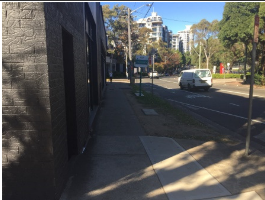
Photo 5.1.2 View of western side of building on site, adjacent to Herbert Street
