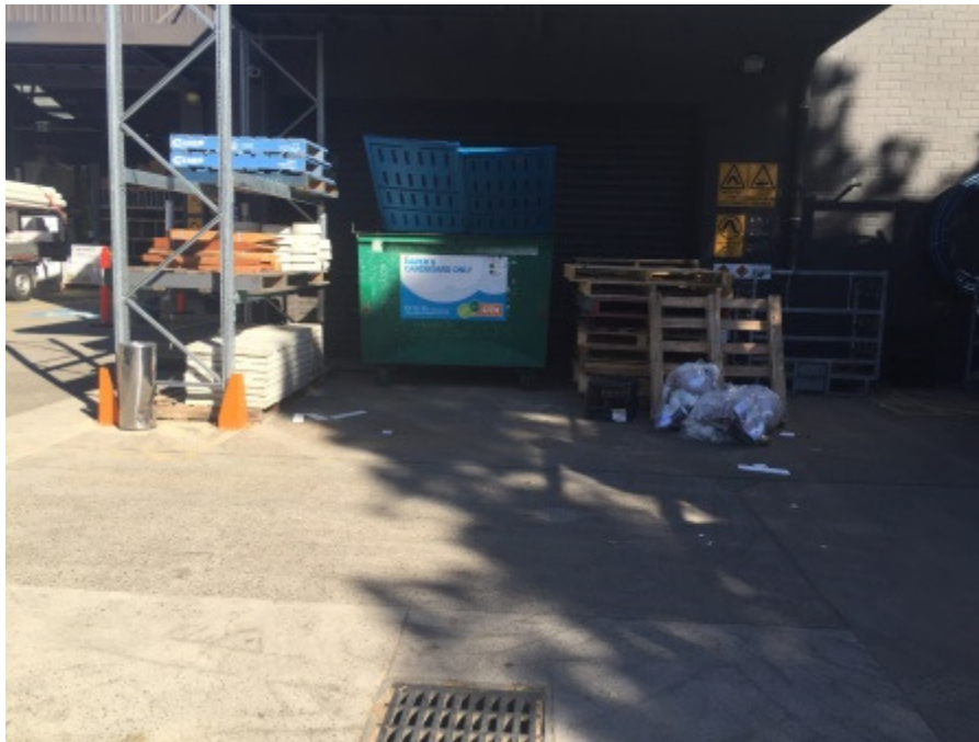
Photo 5.1.6 Eastern side of warehouse building, with access to warehouse and showroom
